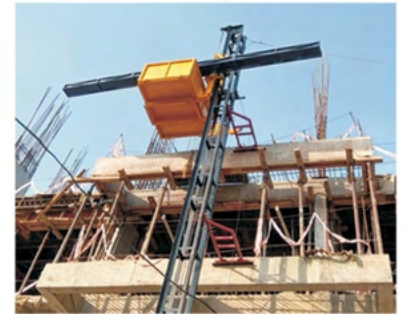
MFH - CMAC Rambo with Rebar Carrier, Delhi
