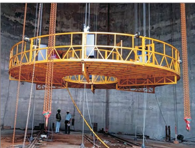
Chimney SRP, Mumbai
