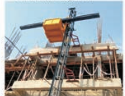
MFH - CMAC Rambo with Rebar Carrier, Delhi
