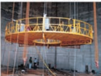
Chimney SRP, Mumbai
