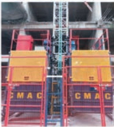
PM Hoist Double Cage, Hyderabad
