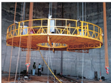
Chimney SRP, Mumbai
