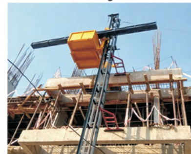
MFH - CMAC Rambo with Rebar Carrier, Delhi
