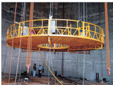
Chimney SRP, Mumbai
