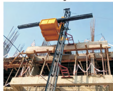
MFH - CMAC Rambo with Rebar Carrier, Delhi
