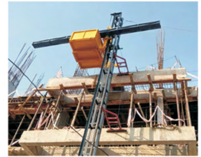
MFH - CMAC Rambo with Rebar Carrier, Delhi
