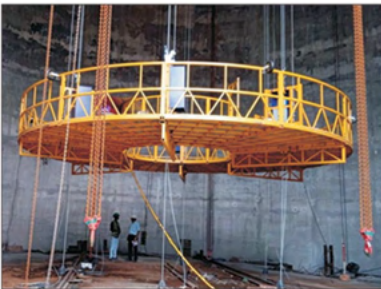
Chimney SRP, Mumbai
