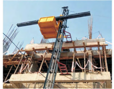
MFH - CMAC Rambo with Rebar Carrier, Delhi
