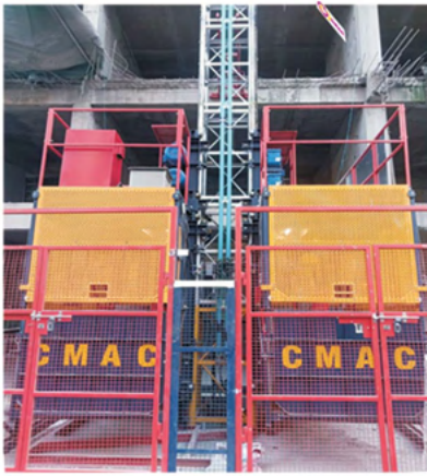
PM Hoist Double Cage, Hyderabad
