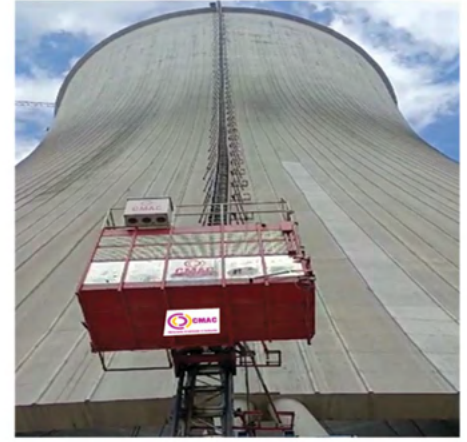
Curved Hoist Bangladesh
