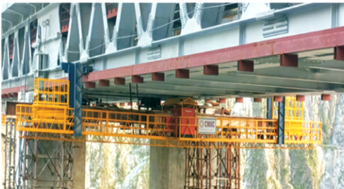
Anji Khad Cable Stayed Bridge Project, Dist.: Reasi, Jammu
