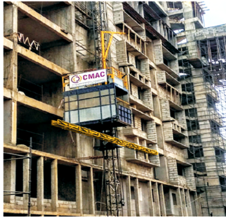
PM Hoist with 12mts Horizontal rebar carrier, Vijayawada
