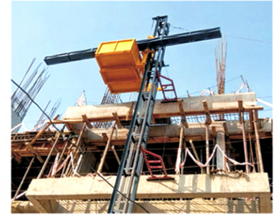
MFH - CMAC Rambo with Rebar Carrier, Delhi
