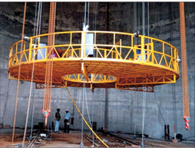
Chimney SRP, Mumbai
